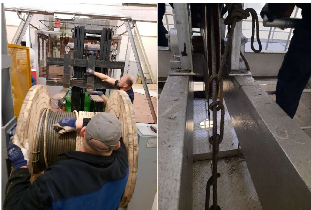
Figure 20 - Replacing the rope in the ventilation building.
