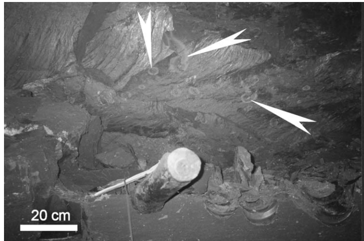
Fig. 12. Oxidation at a depth of 2 m behind the Starting Chamber. The oxidation marks are formed around small pyrite nodules present in the clay.
