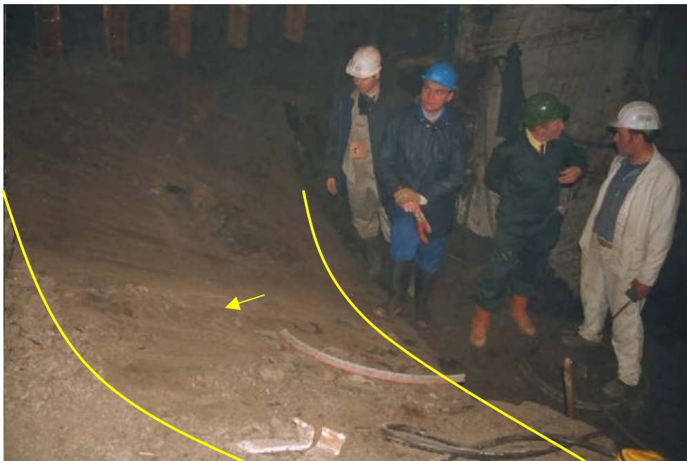
Figure 6: A slip plane observed during the excavation of the starting room
