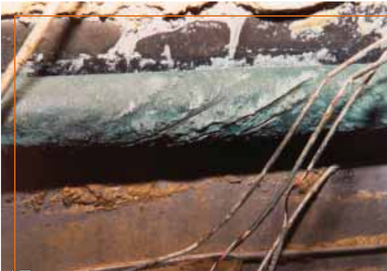
Figures 17: galvanic or electrolytic corrosion on the total length of hydration tube # 07
