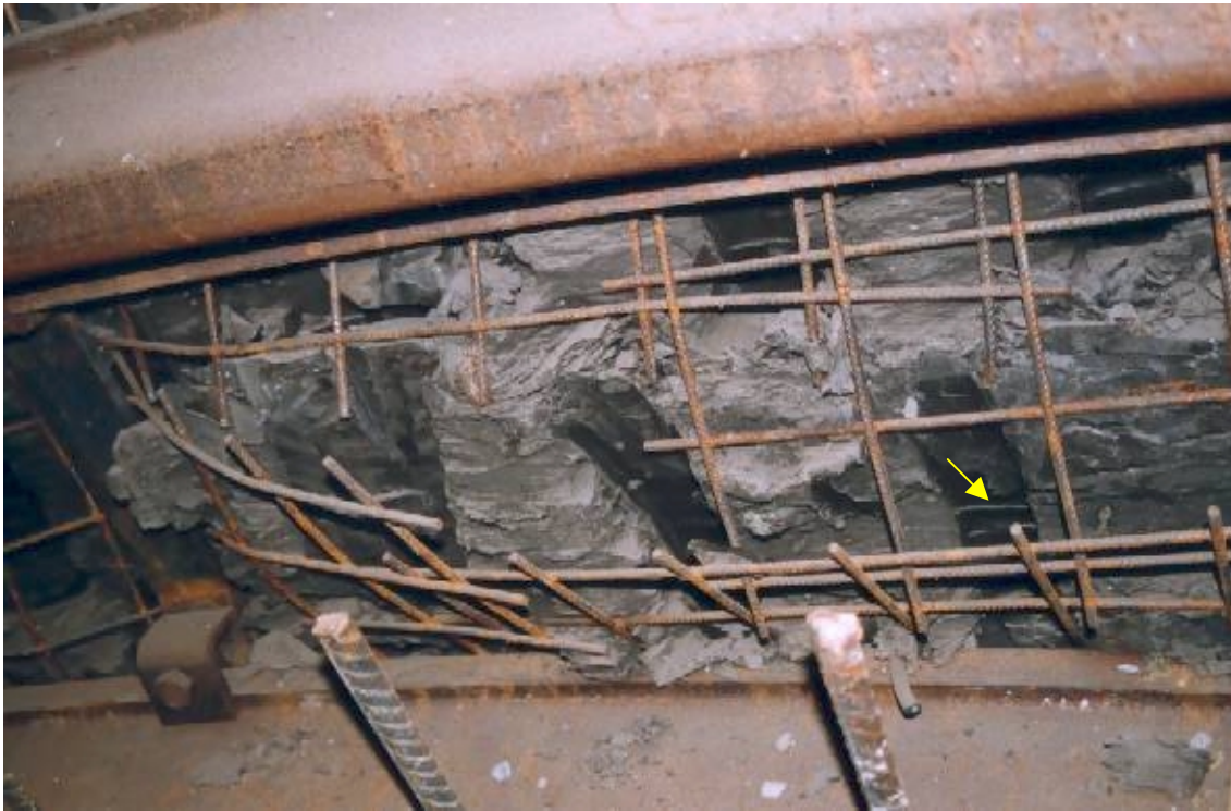
Picture 3: Degraded rock on the lateral excavated wall of the second shaft (1998)
