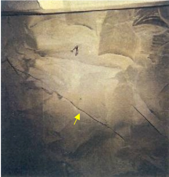
Picture 1: Fractures observed during the excavation of the Test Drift (1987) – East lateral wall
