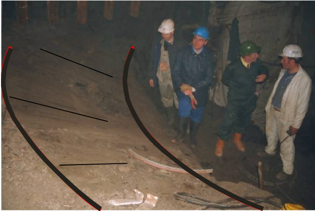
Fig. 4. View of the fracture surface in the South starting chamber (the thick black curves visualise the trace of horizontal planes on the fracture surface).
